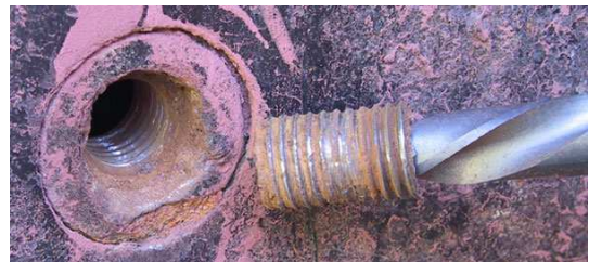
Fig-27 Broken thread
